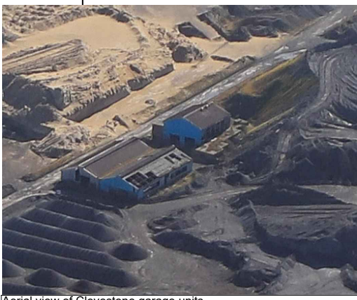
Aerial view of Clevestone garage units
