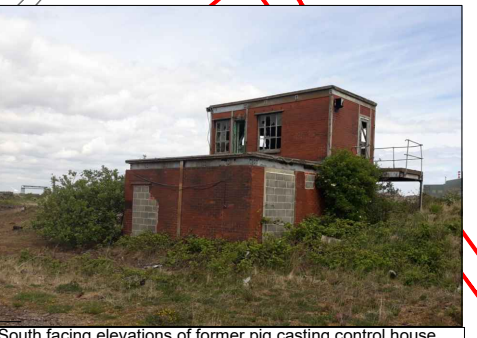
South facing elevations of former pig casting control house
