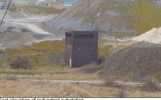
East elevation of redundant substation
